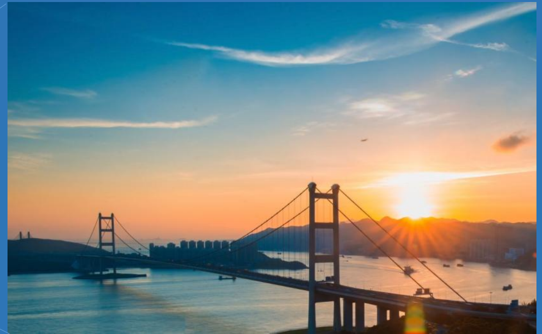
Tsing Ma Bridge: Air draft limitation- 53.0m
